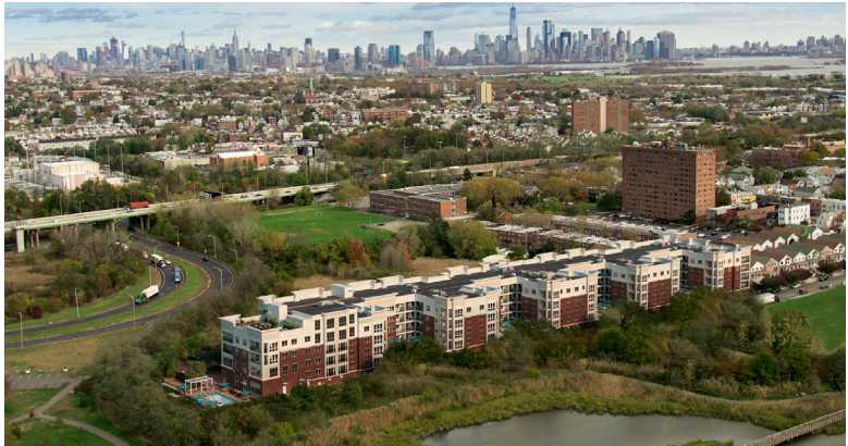
Our Philadelphia team provided a $44 million construction loan to develop a 220 unit luxury multifamily apartment community known as The Woodmont Bay Club in Bayonne, NJ (Hudson Waterfront submarket).
